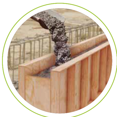
Concrete forming.
