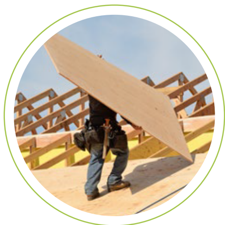
Partition walls, flooring, ceilings and sheathing.
